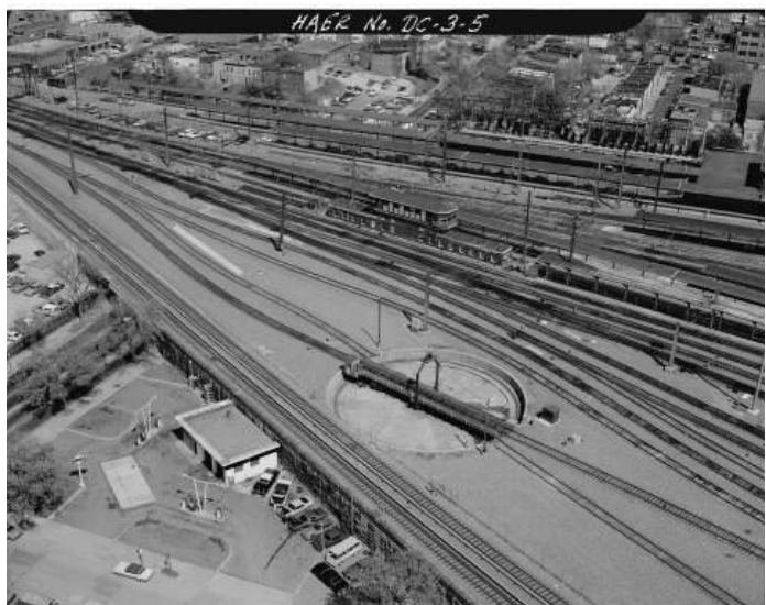
Aerial Photograph, Union Station Turntable, 1977
